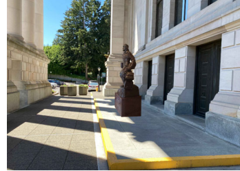
Location 3 South portico Exterior existing slab
