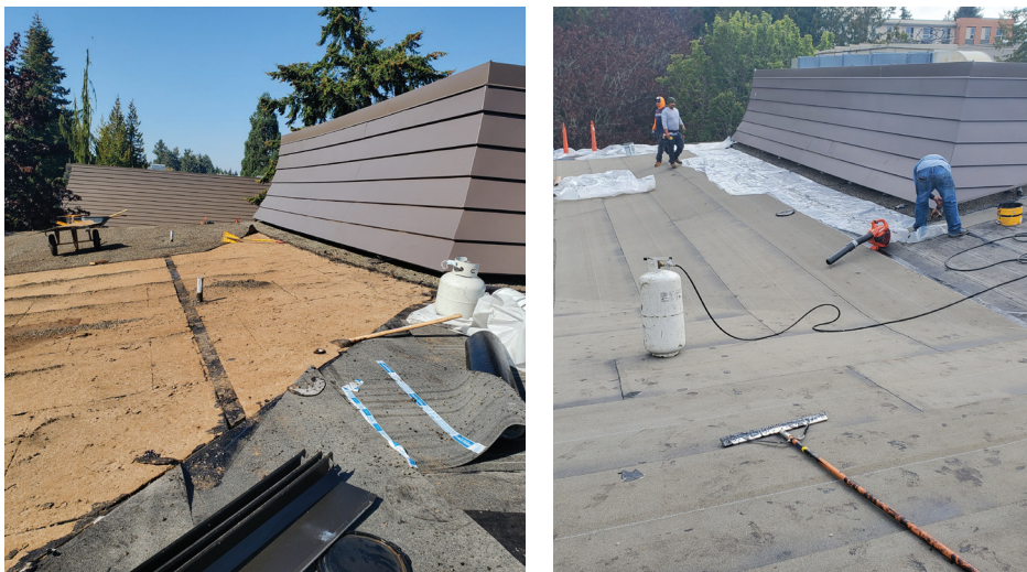
Sequence photos of the 5000 Building Membrane Re-roof
