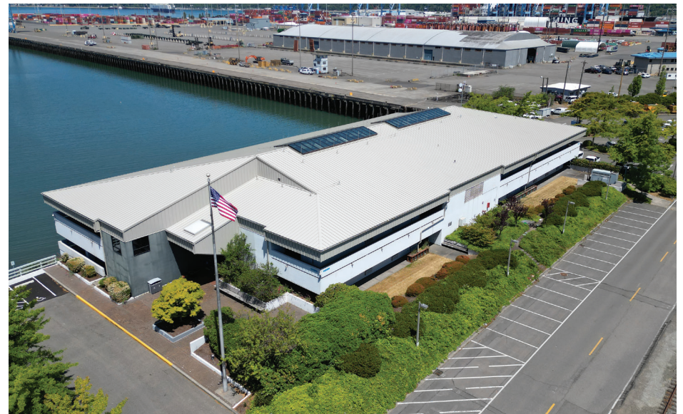
Admin Building's new standing seam metal roof
