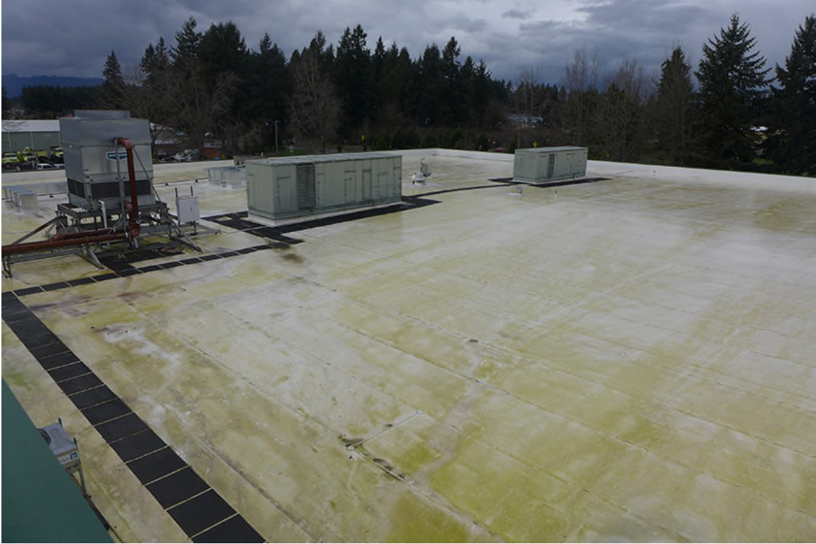
Low Bay Roof PHOTOGRAPH 3
