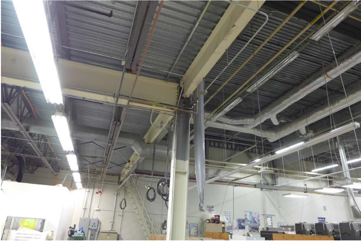
Underside of Mezzanine PHOTOGRAPH 9
