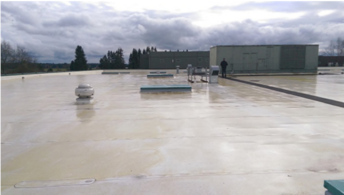
High Bay Roof PHOTOGRAPH 4
