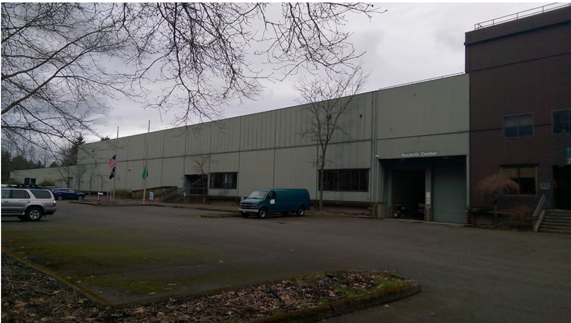
High Bay Section of Modular Building (Isabella Bush Building at right) PHOTOGRAPH 2
