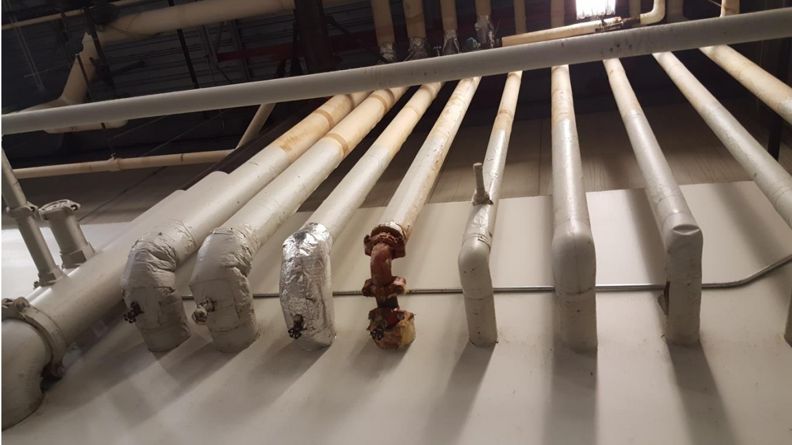
Abandoned Steam Piping PHOTOGRAPH 14
