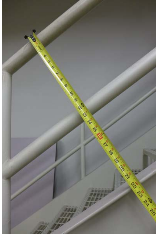
Mezzanine Stair Railing PHOTOGRAPH 13
