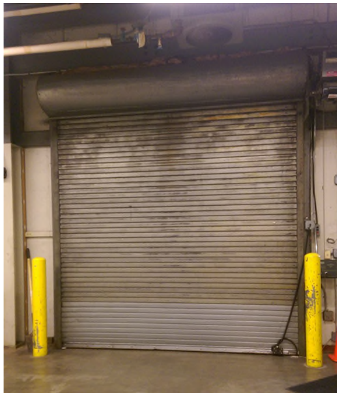
Overhead Rolling Door PHOTOGRAPH 20
