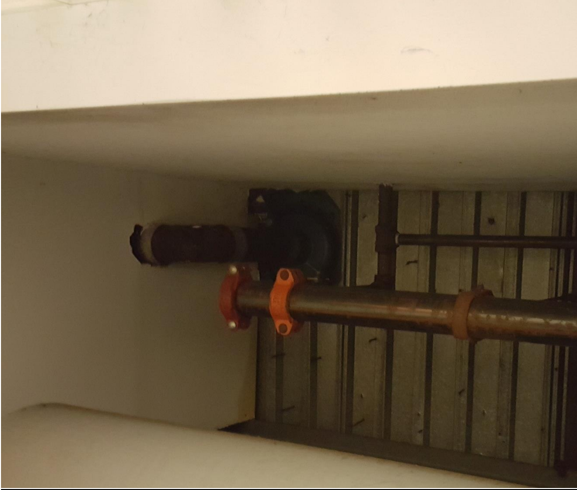
Roof Drain and Drain Piping, Uninsulated PHOTOGRAPH 24
