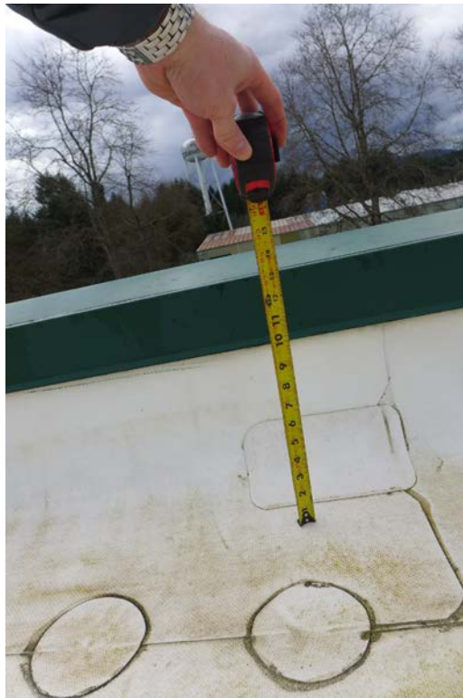
Parapet From Roof (at roof "ridge") PHOTOGRAPH 1
