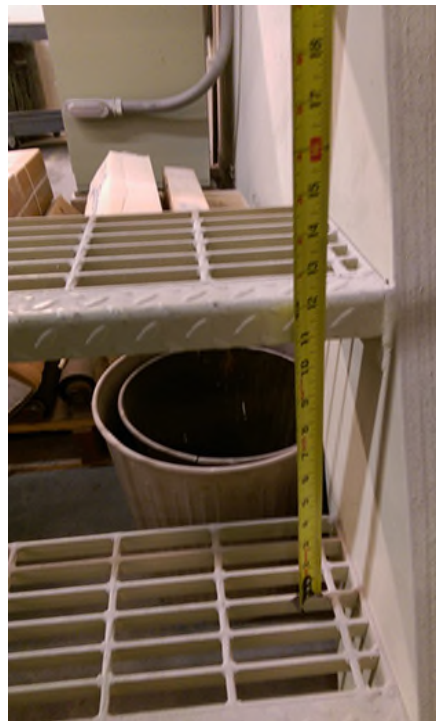
Riser Dimension at Ship's Ladder PHOTOGRAPH 22
