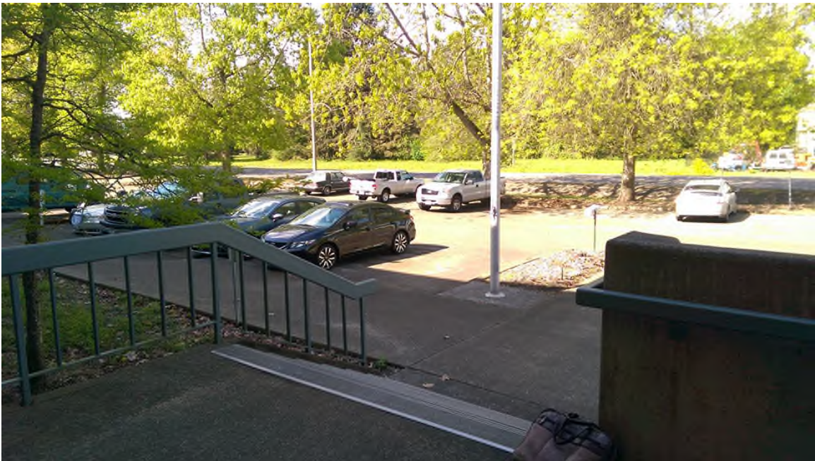
Guardrail at Entry PHOTOGRAPH 24
