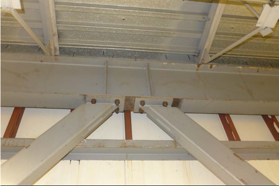
Typical Brace/Beam Connection PHOTOGRAPH 15
