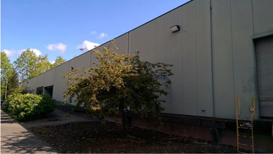
Low Bay Section of Modular Building PHOTOGRAPH 1
