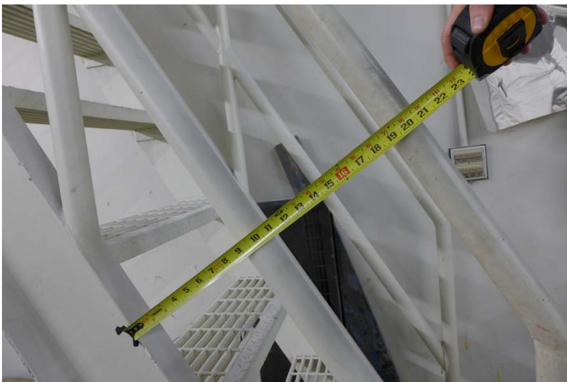
Mezzanine Ships Ladder Railing Detail PHOTOGRAPH 12
