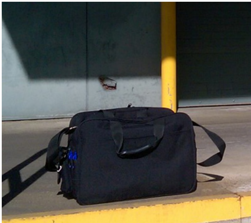
Damaged Panel at Loading Dock PHOTOGRAPH 16
