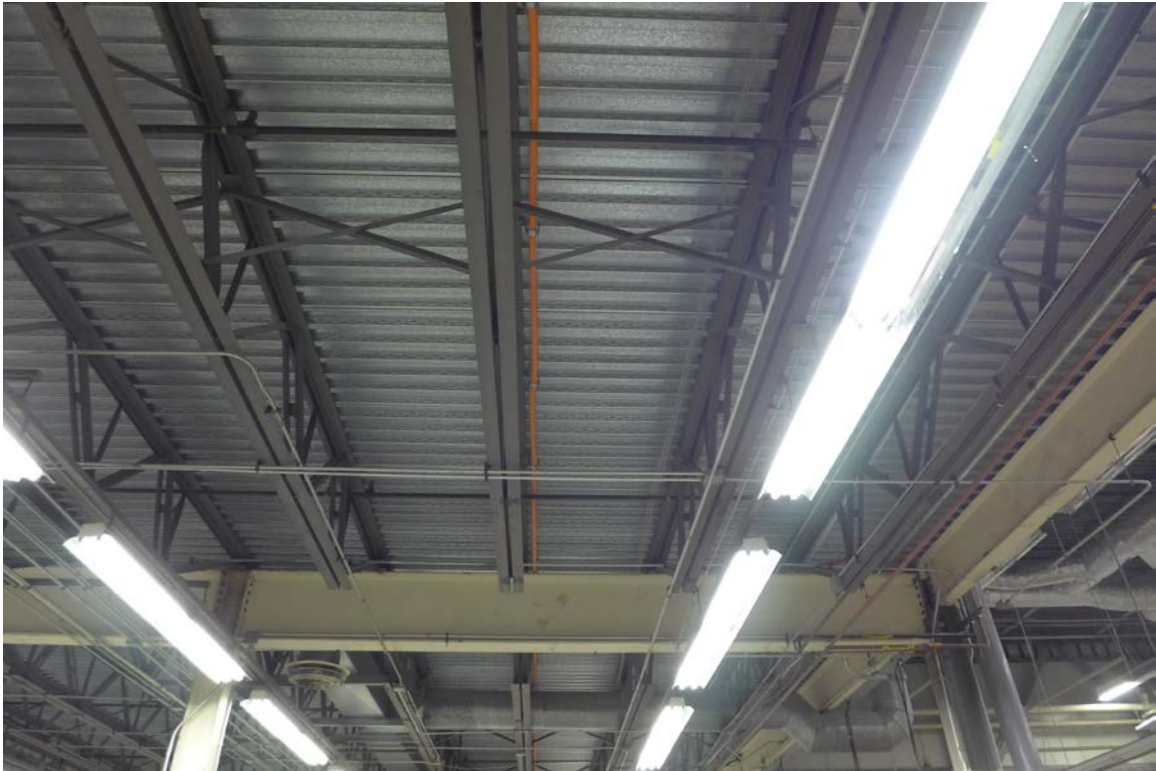
Mezzanine Framing PHOTOGRAPH 10
