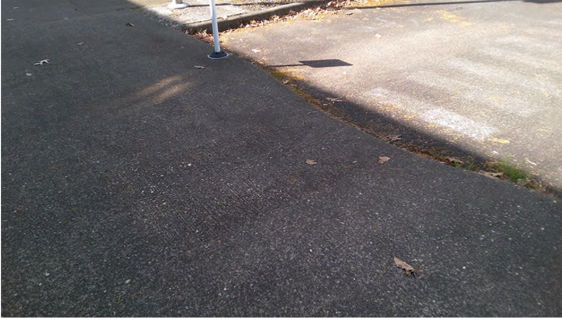
Path of Travel at Vehicular Way PHOTOGRAPH 25
