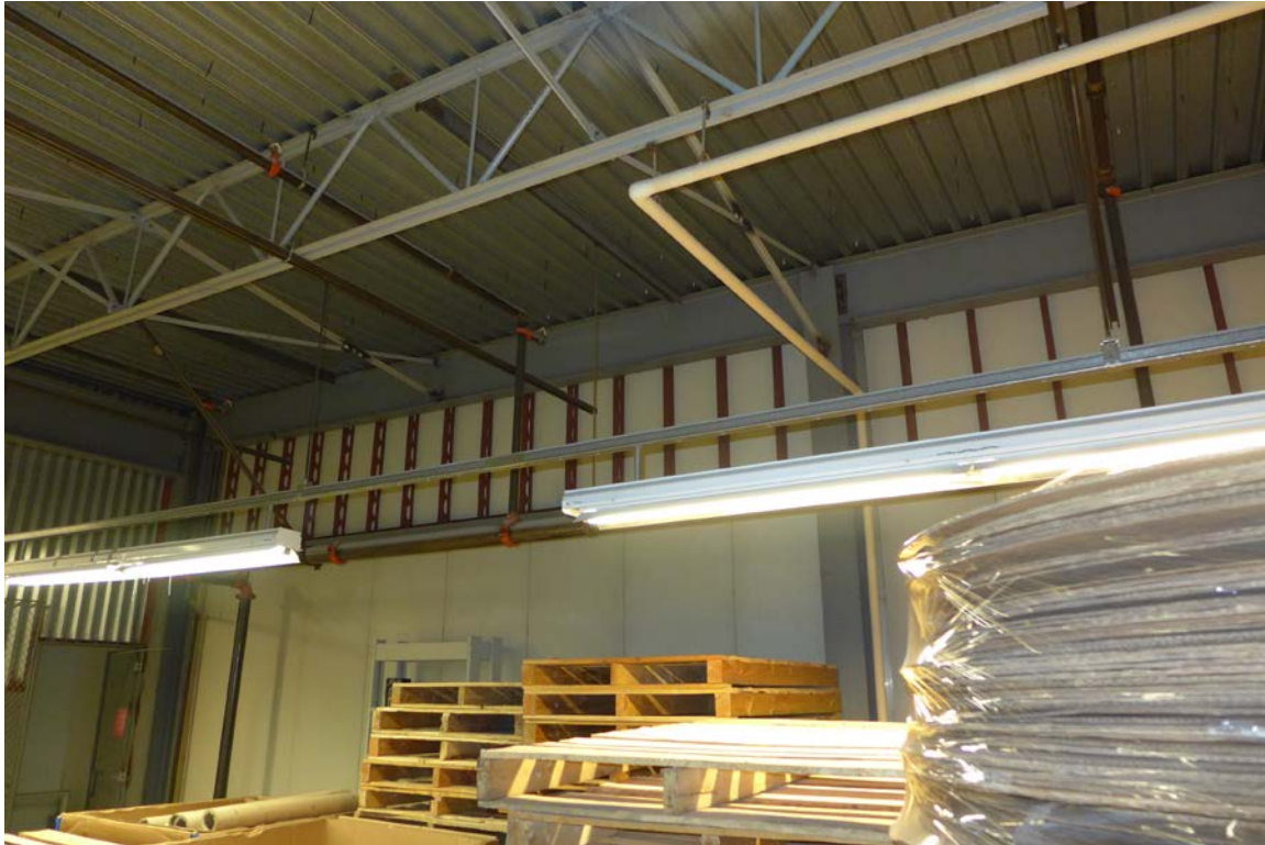
Parapet Base From Interior (from Mezzanine) PHOTOGRAPH 2
