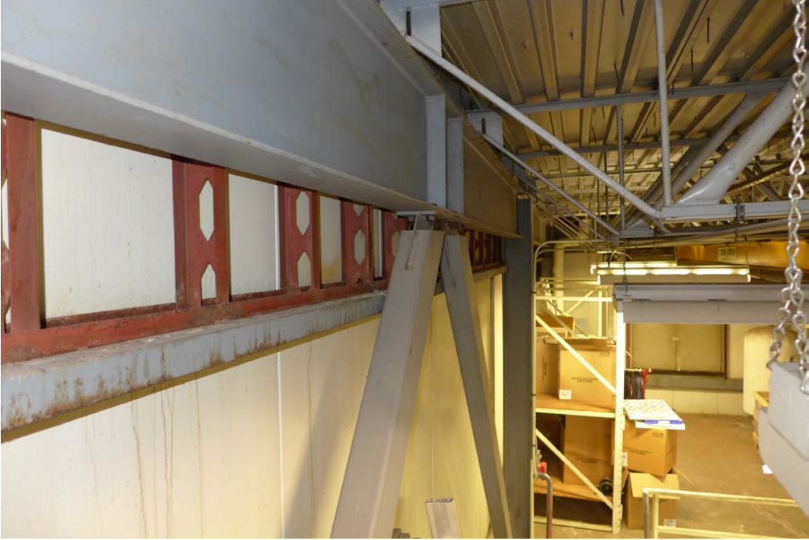
Parapet Base Detail (from roof access) PHOTOGRAPH 3
