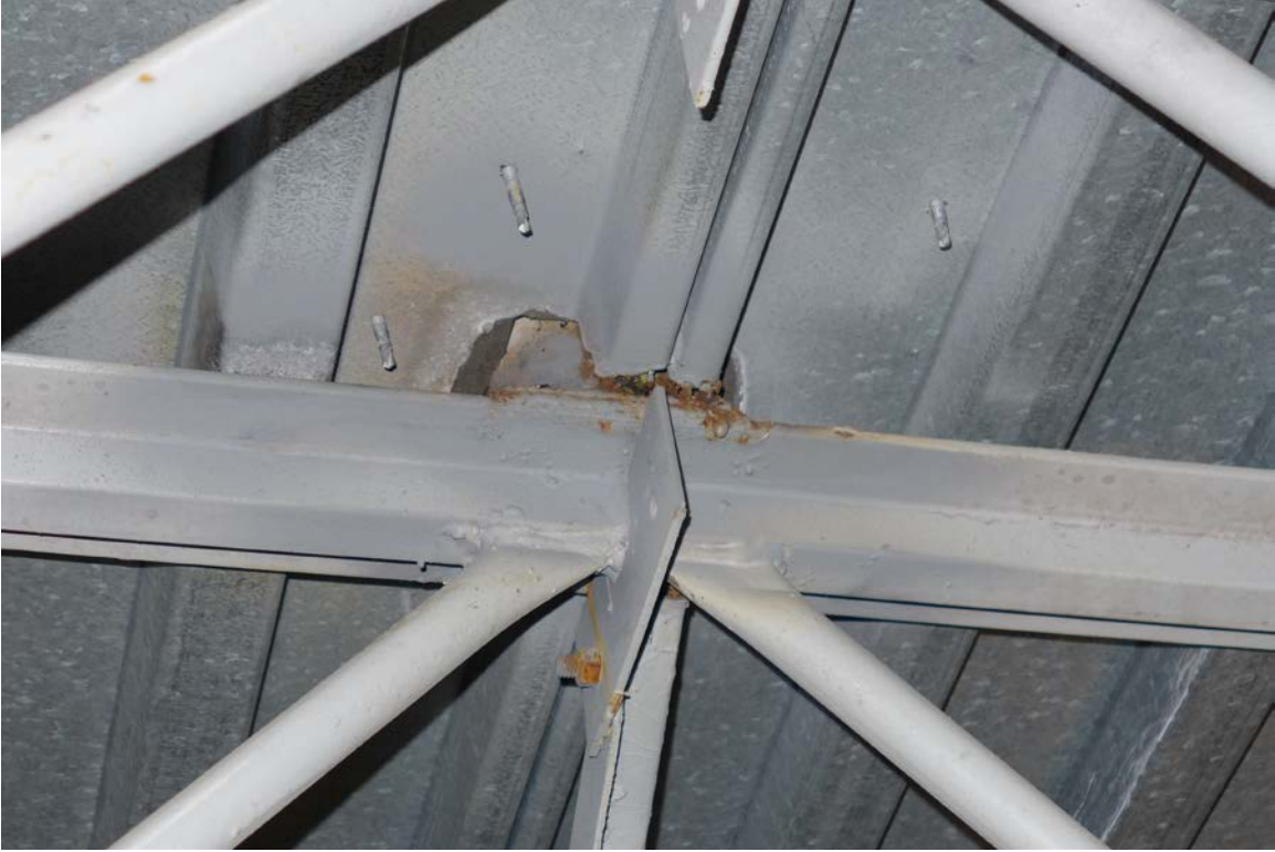
Cooling Tower Support Pipe Connection to Joist Below PHOTOGRAPH 7
