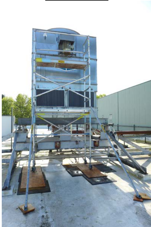
Cooling Tower Scaffolding PHOTOGRAPH 6
