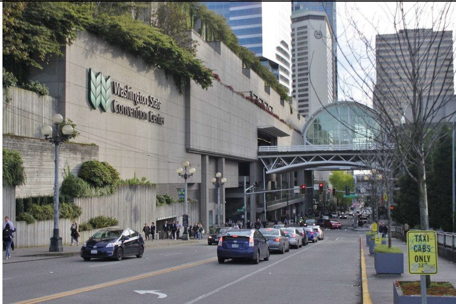
GFRC INSTALLATION: WASHINGTON STATE CONVENTION CENTER, BUILT 1987, 36 YEARS
