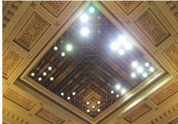
Figure 19: House ceiling laylight, showing downlight configuration
