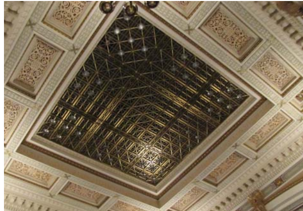
Figure 16: House bronze ceiling laylight
