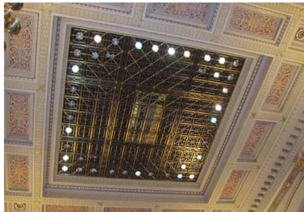
Figure 20: Senate ceiling laylight, showing downlight configuration
