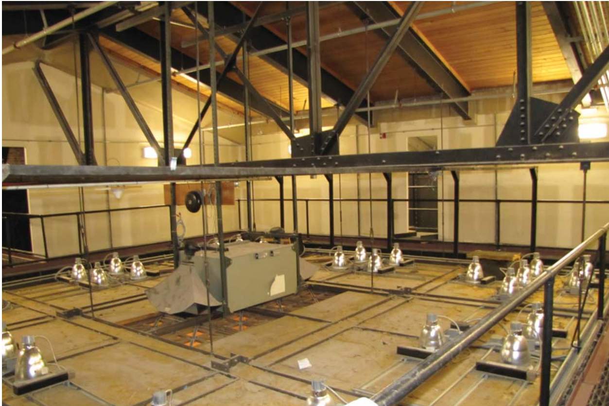
Figure ES05: House skylight attic showing top of bronze ceiling laylight with speaker cluster at the center. A perimeter catwalk provides access.
