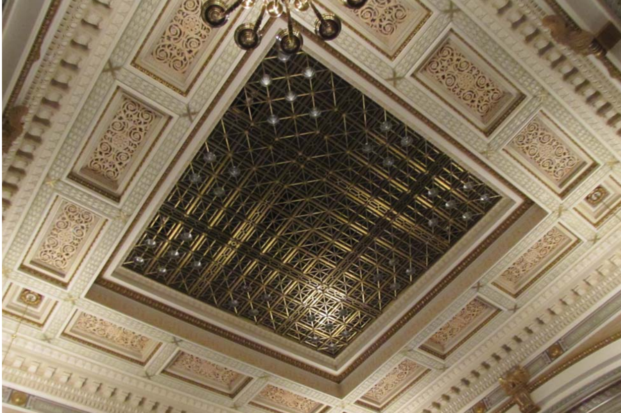
Figure 32: Current ceiling laylight at House Chambers
