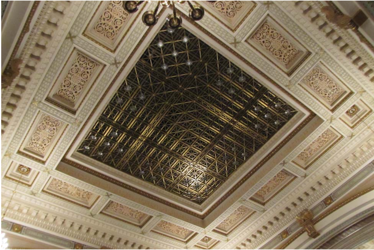
Figure ES03: House bronze ceiling laylight
