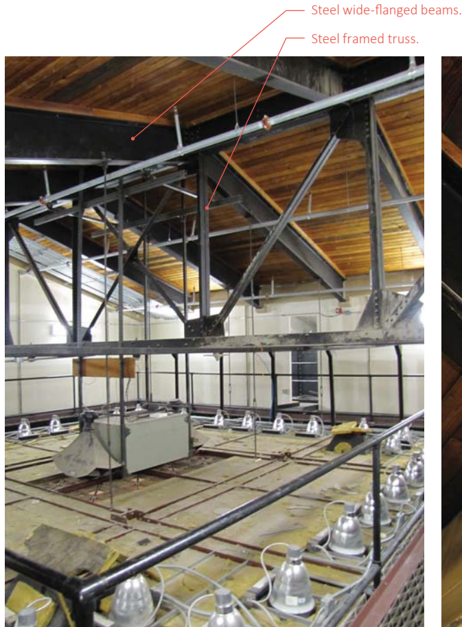
Figure 25: Skylight attic space above the House Chamber (Senate Chamber similar)
