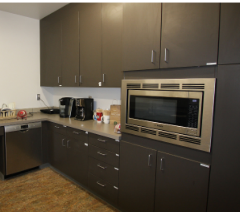
Snohomish Readiness Center Restroom and Kitchen Upgrades - This project included accessibility and gender equity upgrades, HVAC and plumbing systems improvements, and a complete kitchen remodel. From top, original showers used by both males and females within men's restroom; new men's showers; original staff kitchen; and remodeled staff kitchen.
