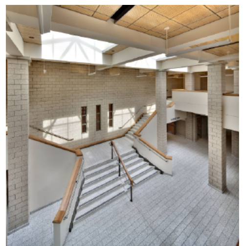
66th TAC Readiness Center: As a demonstration of our commitment to creative solutions that elevate National Guard facilities, knowledge of National Guard Bureau materials allowances allowed Straling Whitehead & Lux Architects to specify wood panels and trim throughout the facility.
