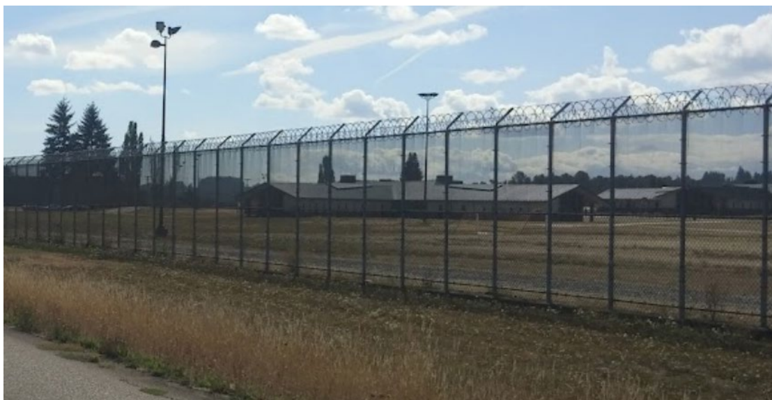
Secure perimeter fence with Concertina wire at Green Hill School (DCYF).
