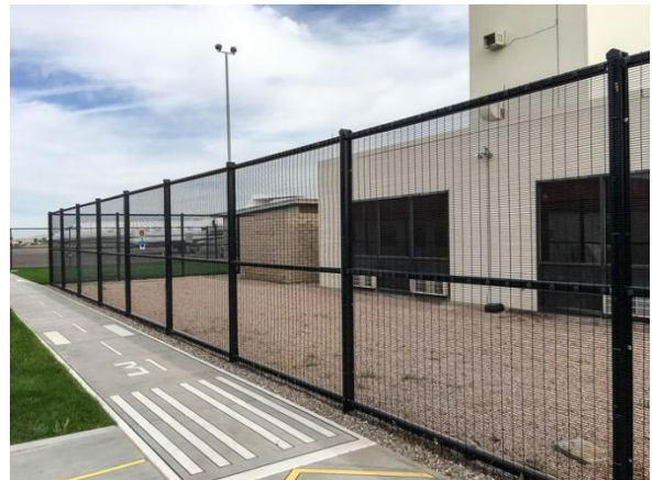
Non-climb welded wire mesh fence system.
