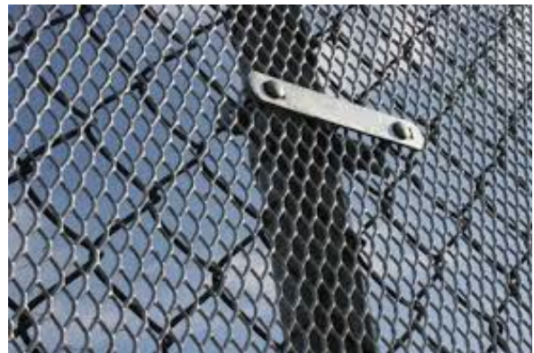
Example of a mini mesh chain link fence fabric in comparison to standard 2-inch chain link.
