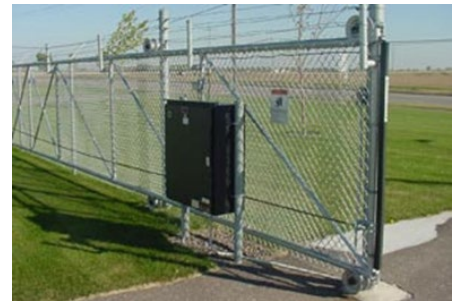
Example of a cantilever sliding chain-link fence.
