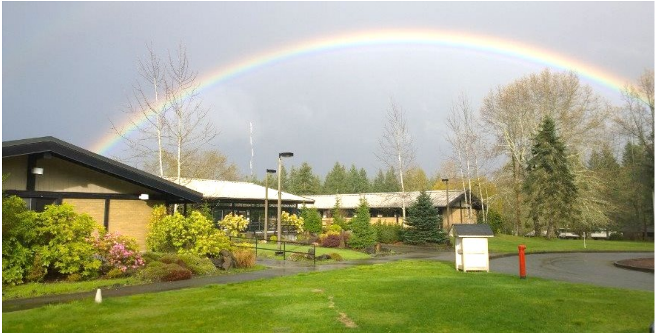
View of the EGCC Health Services, Main Entrance, and Administrative Building from the main visitor parking lot.
