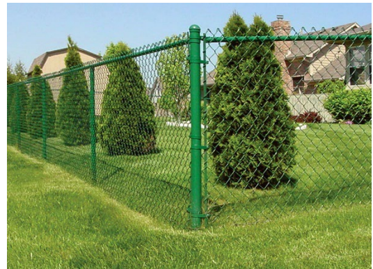
Example of a standard, green-colored vinyl-coated chain link fence.
