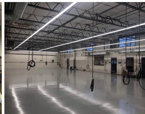
After - Prior to Final Equipment Installation
