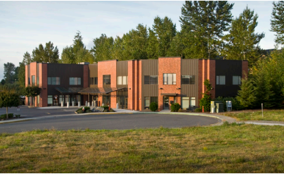
WCC - Foundation Building Exterior
