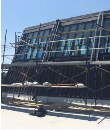
WCC Syre Clerestory - RMC
