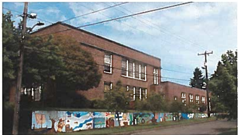
1930 addition eastern façade & retaining wall viewing northwest along 30 th Ave NW.
