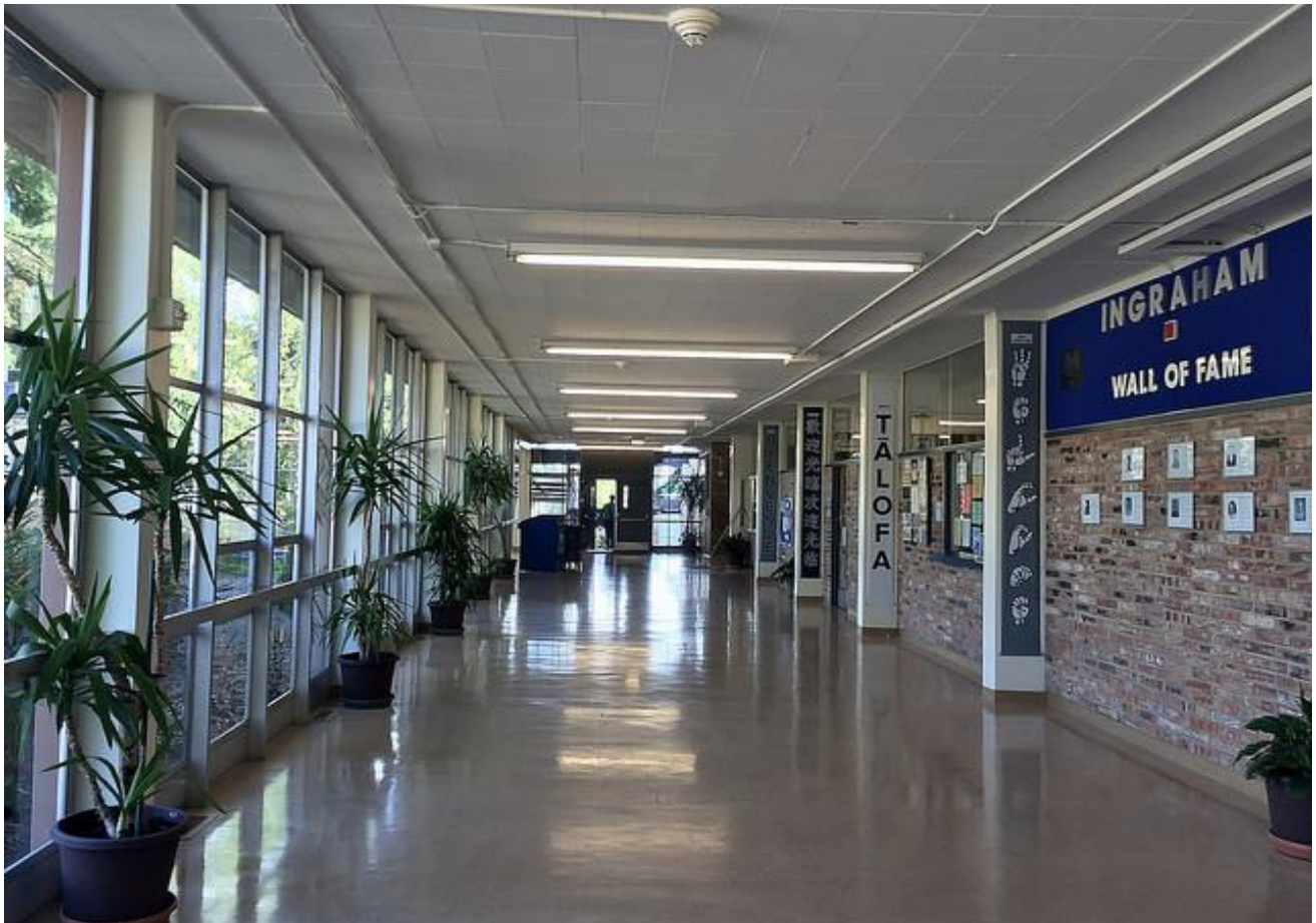
Typical Interior Hallway – Existing Building 100 (circa 1959)
