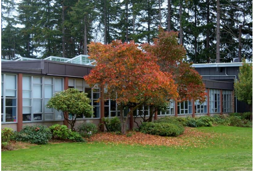
Existing Building 100 - Exterior façade (circa 1959)
