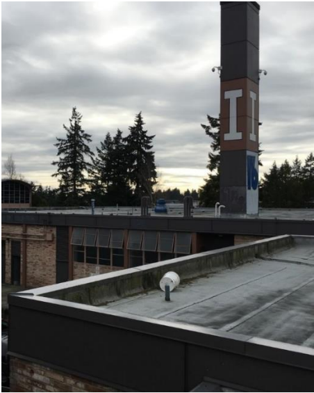
Existing structures and roof (circa 1959)
