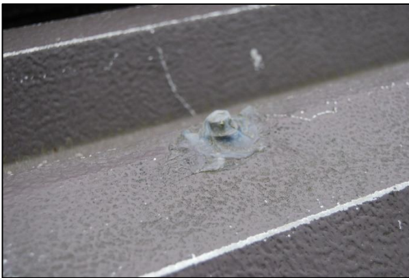
Exposed Fasteners Caulked Over (typ.)
