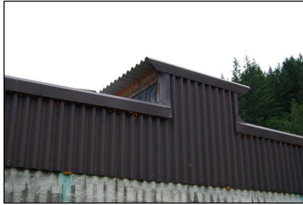
View of Ridge Vent Structure at South Elevation
