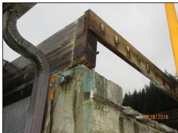
Southwest Corner Panel Removal
