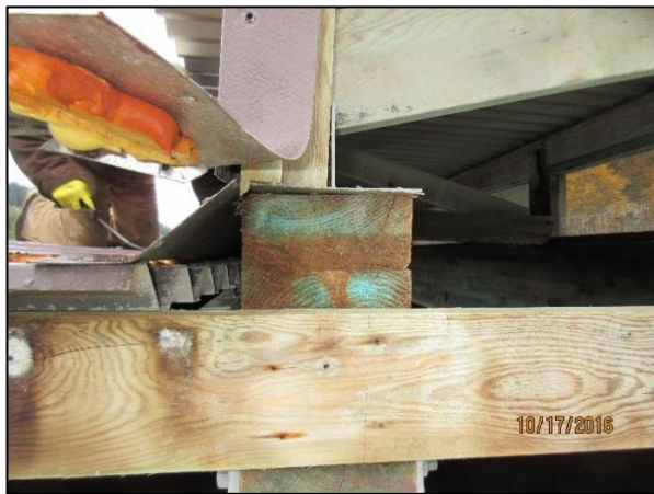
View of Ridge Vent Flashing and Structure Looking North
