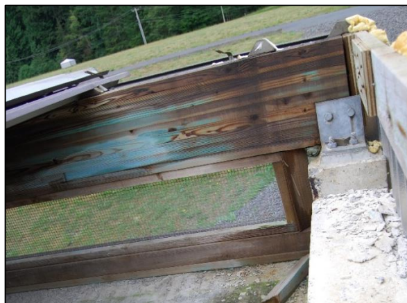
Northwest Corner Panel Removal
