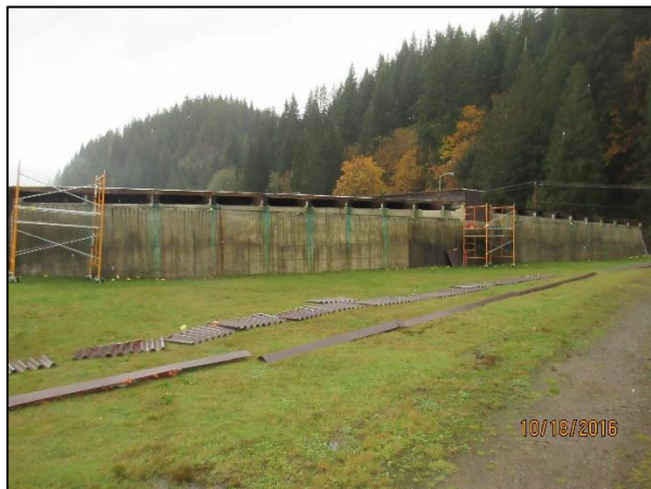
View of South Elevation / Removal of Siding and Flashing
