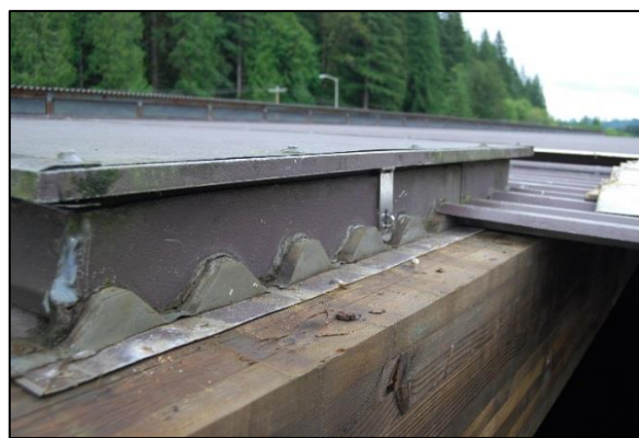
North Panel Removal around Access Hatch
