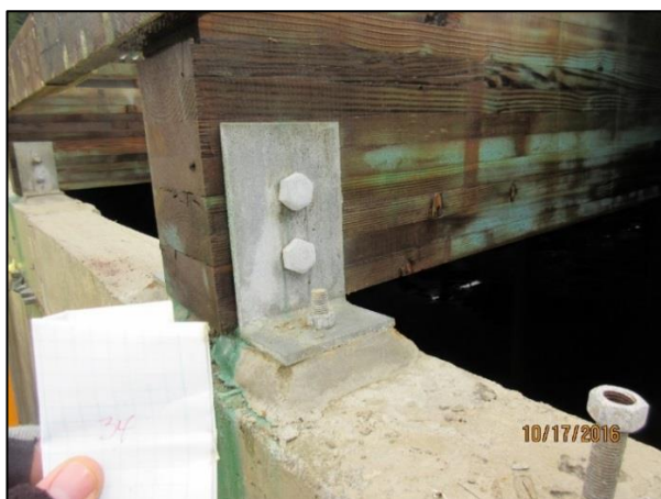
Typical Purlin Support Hanger at Wall
