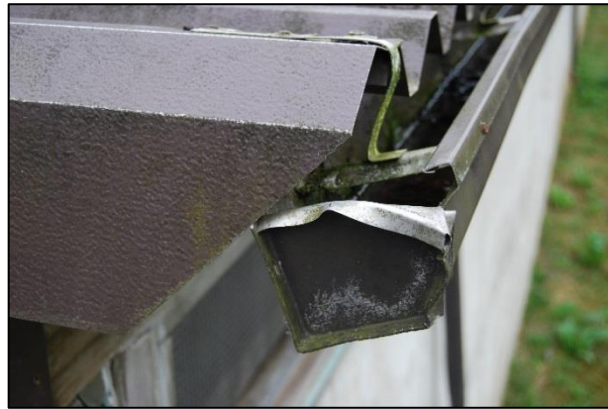
Gutter at Northwest Corner
