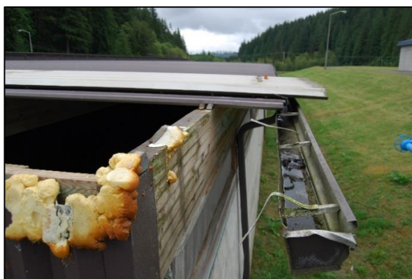
Northwest Corner Panel Removal
