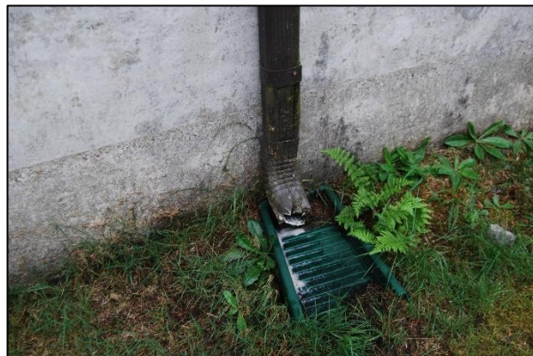
Downspouts and Plastic Splash Blocks (typ.)
