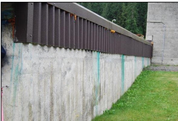
View of North Corner Looking West
