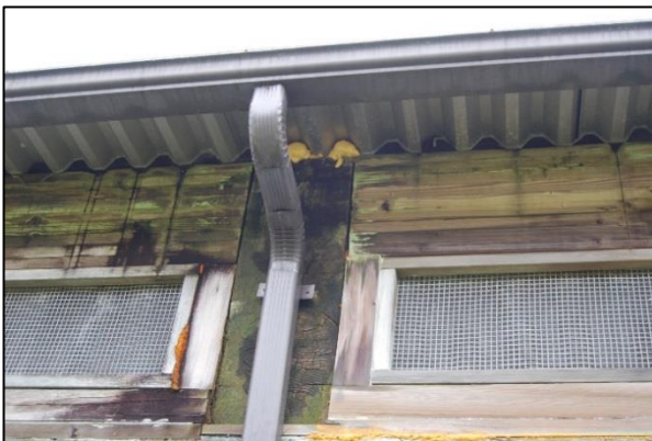
Gutter and Downspout Attached to Posts
