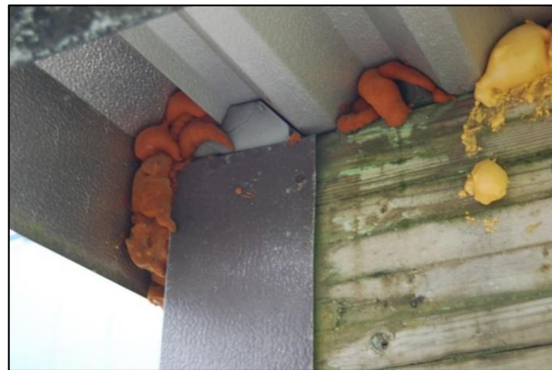
Foam Eave Filler/Spray Polyurethane Foam (typ.)
