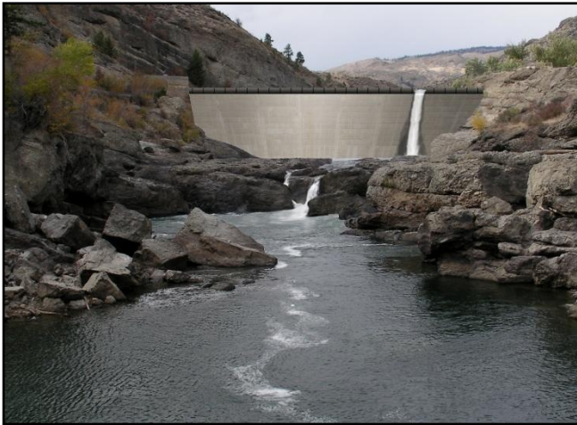
Figure 17. Simulated photo of 30 cfs in "thin stream" over Dam Falls and 30 cfs over Similkameen Falls.
