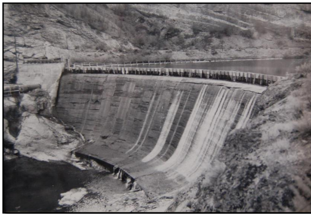
Figure 7. Dam Falls with unknown low (leakage) flow from 1950s (from Similkameen River Trail Facebook Page).
