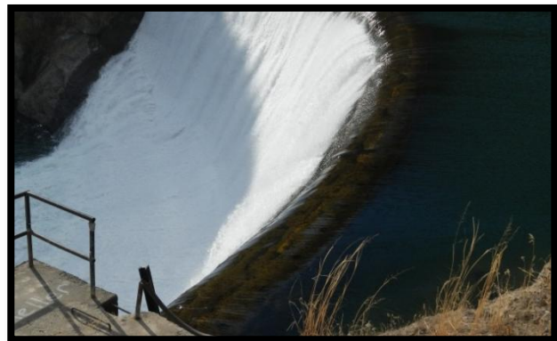
Figure 21. The Dam Falls at 700 cfs showing nappe separation (where falling water becomes aerated).
