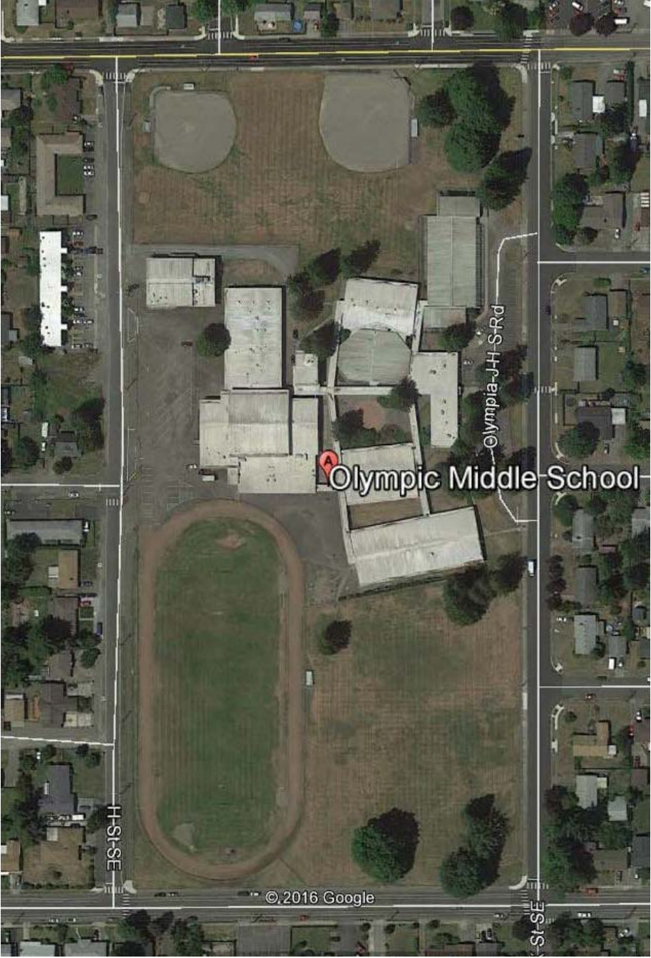
Figure 2 – Existing Olympic Middle School Site Aerial
