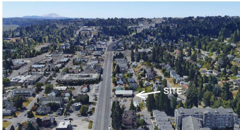
View looking south along Rucker
