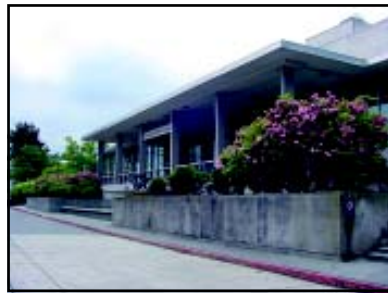
Fig. 3.1.11 2002 photograph of the northwest planter. Photograph by Artifacts Consulting, Inc.
