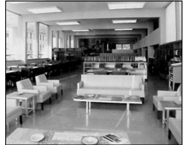
Fig. 2.2.16 Ca 1959 photograph looking east through the low frontal volume of the Library. Photograph courtesy of the Washington State Library.
