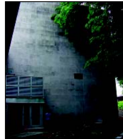
Fig. 3.1.6 2002 photograph of west facade. Photograph by Artifacts Consulting, Inc.
