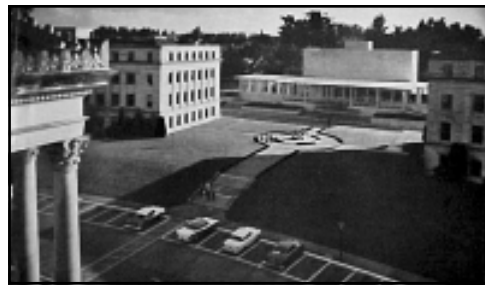
Fig. 2.2.4 Ca 1959 photograph taken from the upper portion of the Legislative Building looking southeast at the Library. Photograph courtesy of the Washington State Library.
