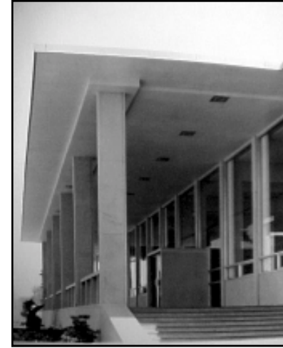
Fig. 2.2.13 Ca 1959 photograph looking east through the portico at the entry vestibule. Photograph courtesy of the Washington State Library.
