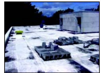
Fig. 3.1.9 2002 photograph of the stack roof. Photograph by Artifacts Consulting, Inc.
