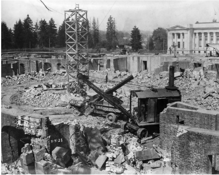
Photo 1- Removal of original Capitol building foundation, 1923. On file at: https://www.sos.wa.gov/legacy/legbuilding/construction.aspx
