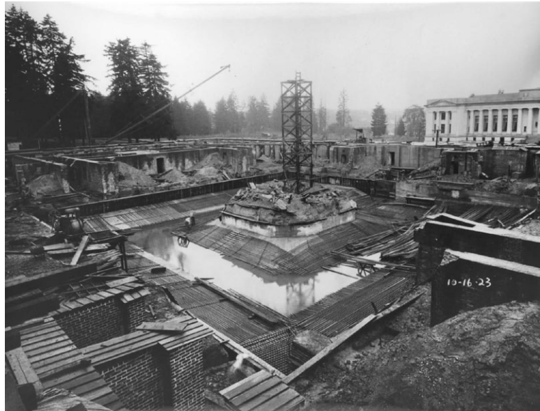
Photo 2- Installation of new Capitol Building foundation, 1923. On file at: https://www.sos.wa.gov/legacy/legbuilding/construction.aspx
